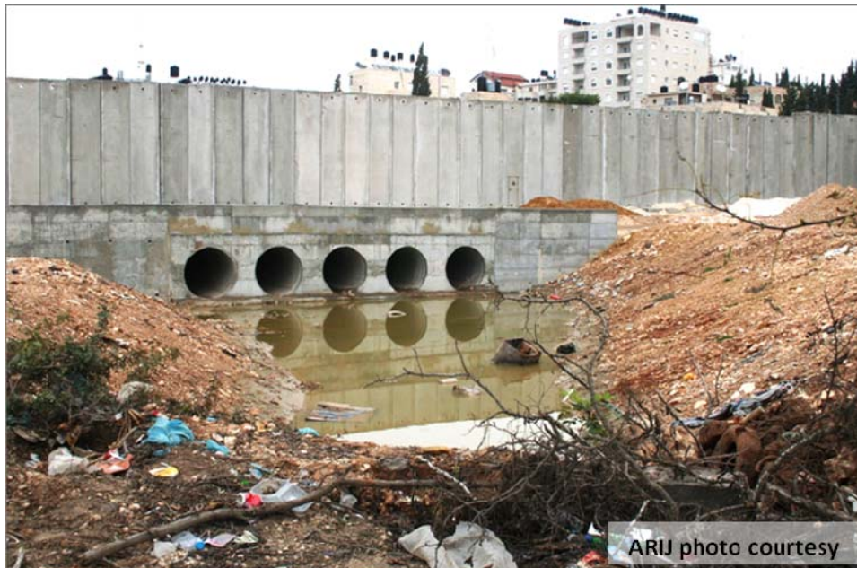
Photo 2: The Wall constructed above the sewage lines
