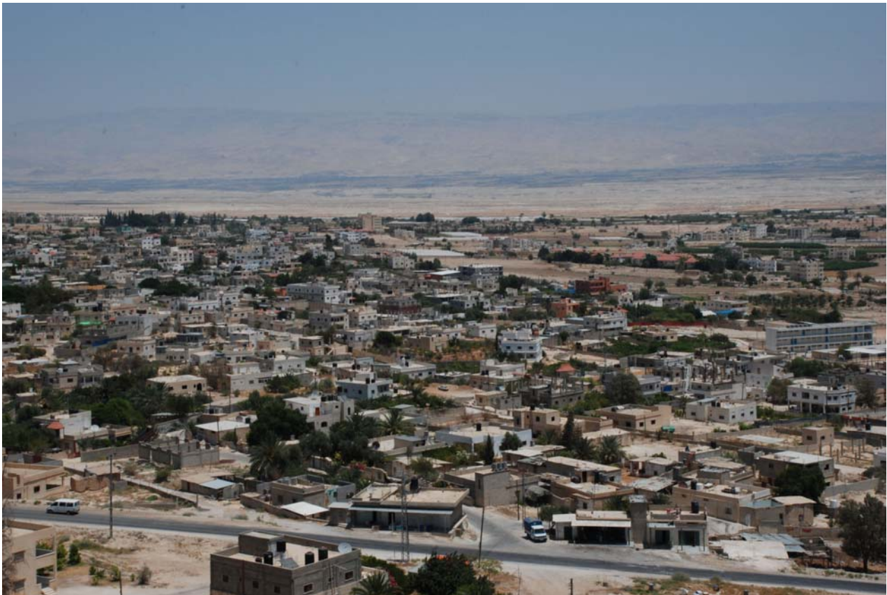
Photo 1: General view of the residential area of Jericho City
